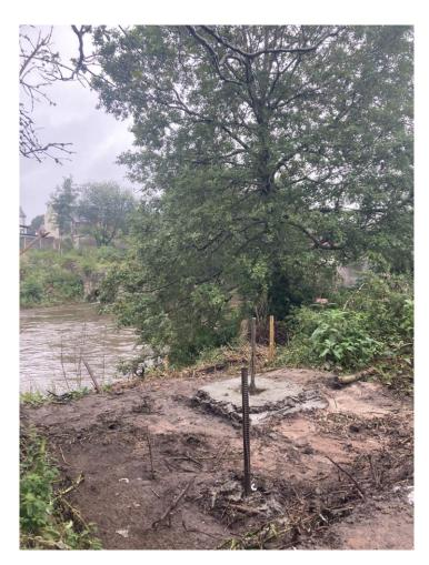
Over the summer ground investigations and soil nail tests were carried out on the riverbank to identify if this intervention is appropriate in this location.
