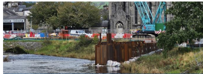
Temporary sheet piled cofferdam creating a dry working area for the construction of the new Stock Beck outfall.
