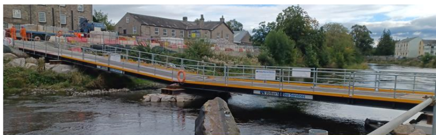
Temporary in-river bridge crossing and working platform
