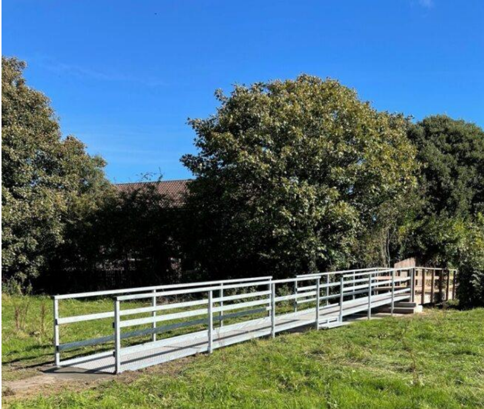
Image: Temporary approach ramp set to be replaced.
