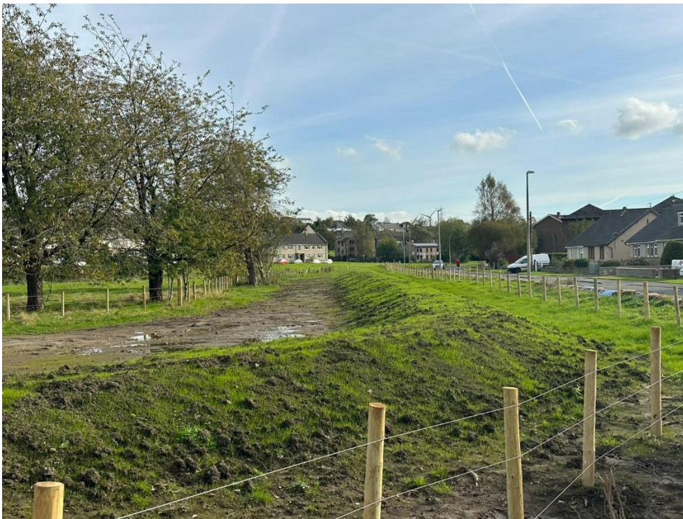
Image: View of completed embankment, with grass beginning to establish.
