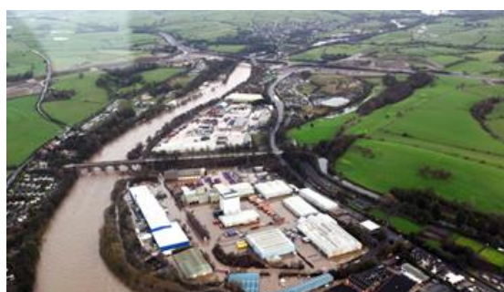
The Caton Road scheme in Lancaster benefits business and infrastructure rather than residential properties so did not attract much GiA funding. It was only made possible with a £2m contribution from the RFCC's Local Levy fund.
