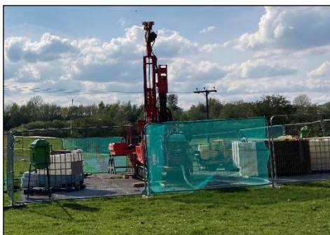
Example rig drilling a borehole to install a monitoring well
