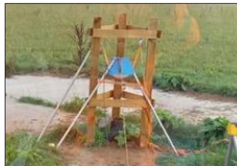
Example monitoring well set-up
