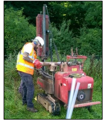
Window sample rig
