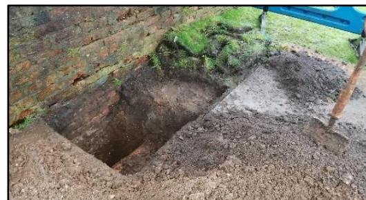
A hand dug trial pit
