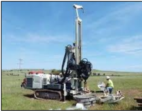
Sonic drilling rig
