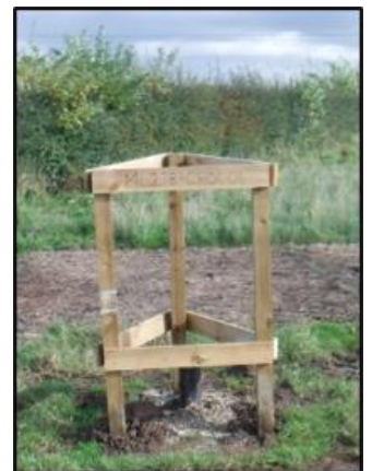
Monitoring installation (land prior to reinstatement)
