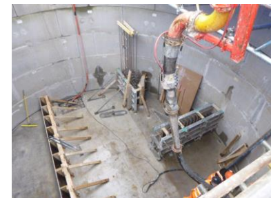
Wet Well Shaft
