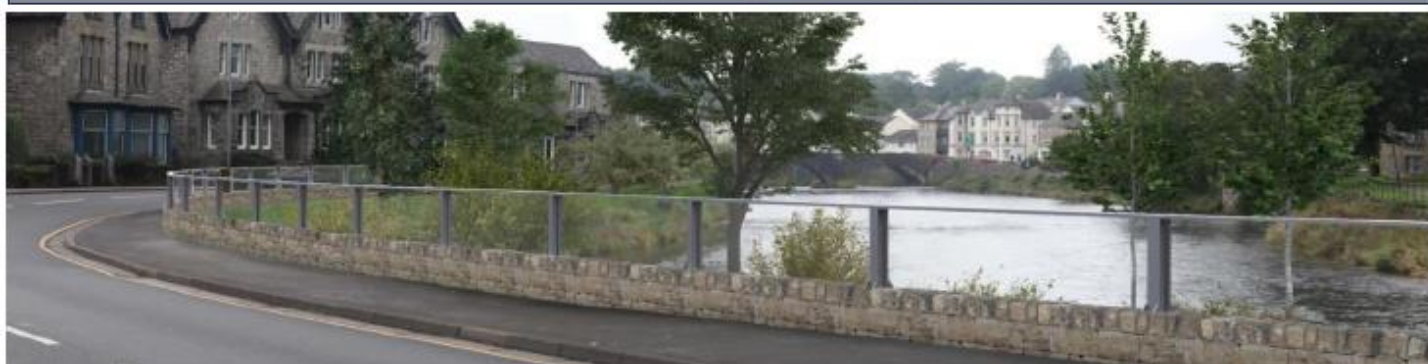
411 metres of glass panelled flood wall retaining riverside views
