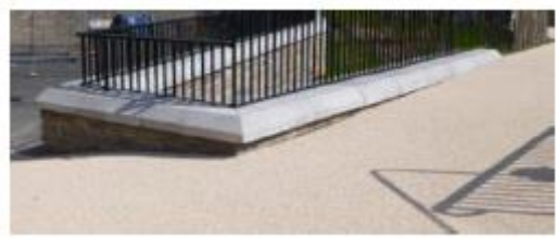
A combination of two coping stone finishes similar to that used at Parish Church.
