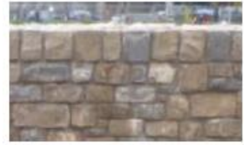
A combination of two coping stone finishes similar to that used at Parish Church.
