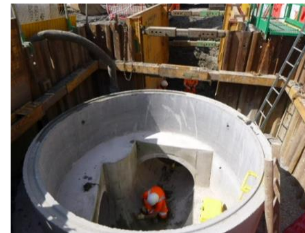
Sewer Diversion – sheet piled dry working area with new sewer pipe
