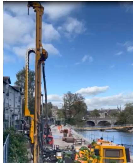
Trial Piling Rig
