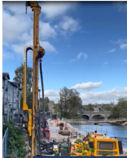
Trial Piling Rig
