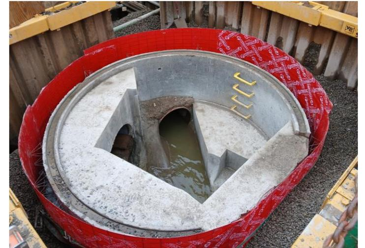
Sewer Diversion – sheet piled dry working area with new sewer pipe
