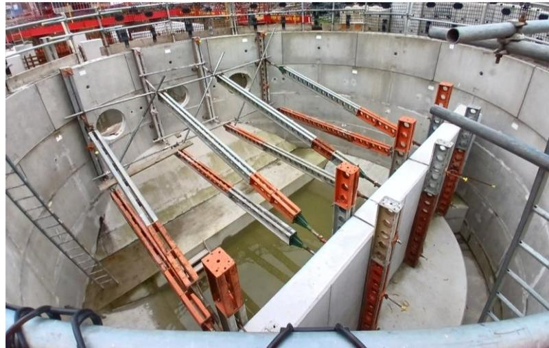
Wet Well Shaft – Underground housing of the pumps for Stock Beck
