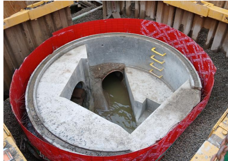
Sewer Diversion – sheet piled dry working area with new sewer pipe
