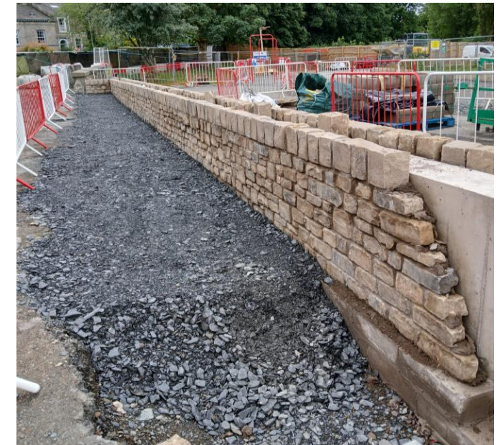
Floodwall along St Georges walk in Construction
