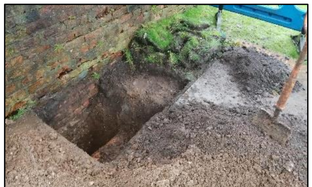
A hand dug trial pit
