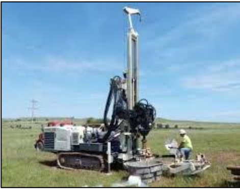
Sonic drilling rig
