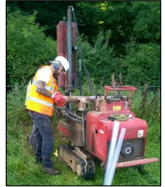
Window sample rig
