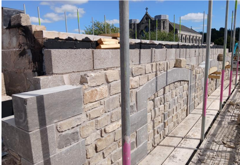
Motor Control Centre Building – Housing for all the electrical equipment for the Stock Beck pumps
