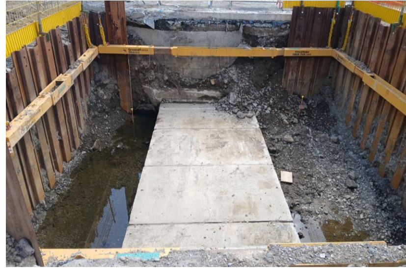
Sewer Diversion – Sheet piled area for the underpass chamber once Stock beck culvert is removed
