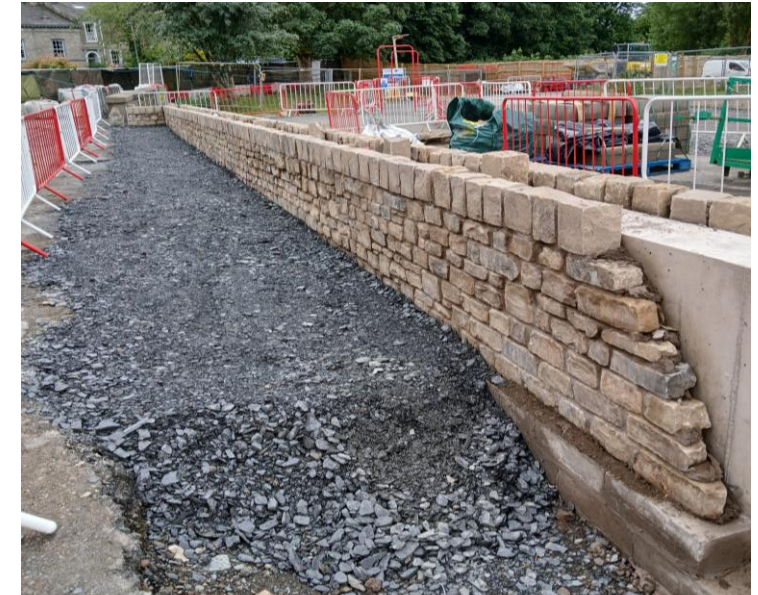
Floodwall along St Georges walk in Construction
