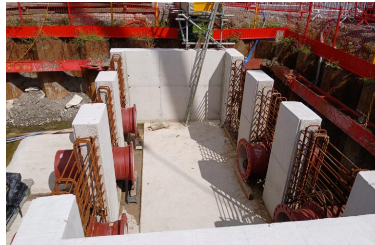
Valve chamber – Holding the pipe valves that pump Stock Beck onwards to the outfall
