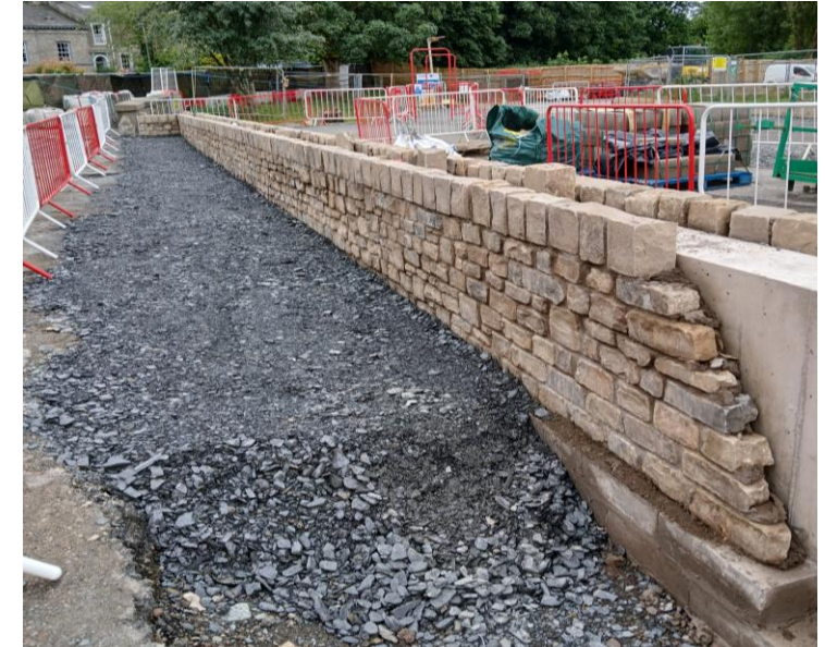
Floodwall along St Georges walk in Construction
