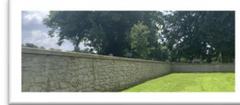
Waterside Flats Flood defence wall in vicinity of residential flats. Natural stone cladding to outward facing wall with imprinted concrete to residential side. Floodgates maintaining pedestrian access to riverside.
