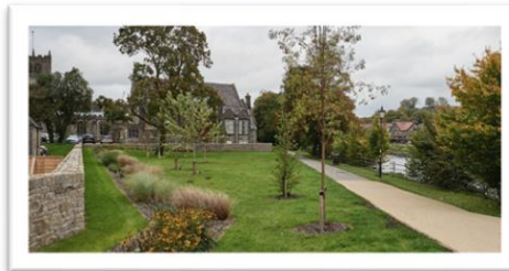
Parish Church frontage Stone clad wall with low sections topped by railing. Access ramp over flood defence linking to Kirkland.
