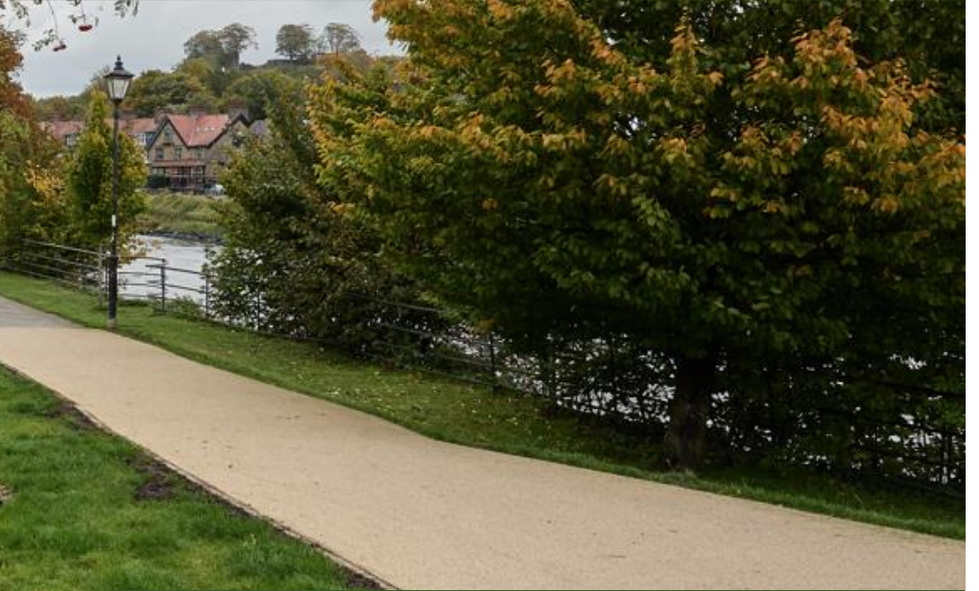
AFTER FLOOD WALL CONSTRUCTION AND LANDSCAPING
