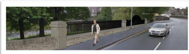
Miller Field Stone faced wall featuring Webster railing design and new riverside footpath.
