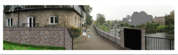
New Road Common Land Stone faced flood defence wall to tie into new footbridge access ramp. Floodgates to maintain public access through open space.
