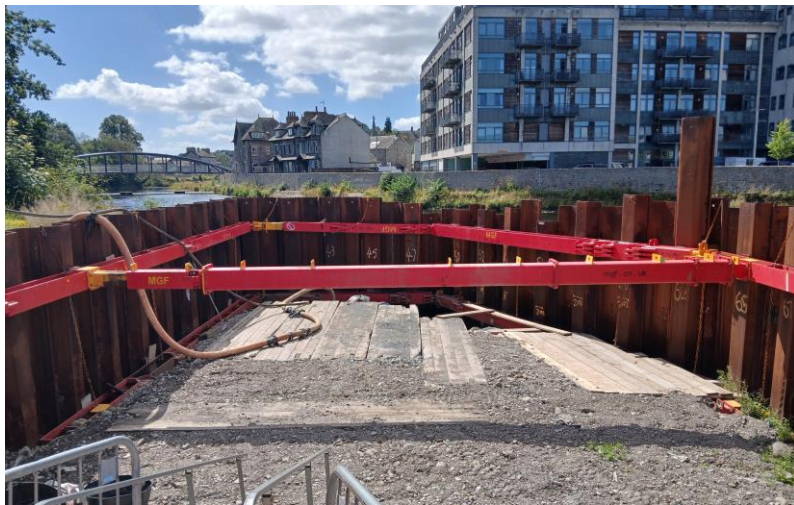
Outfall – The new outfall of Stock Beck into the River Kent.
