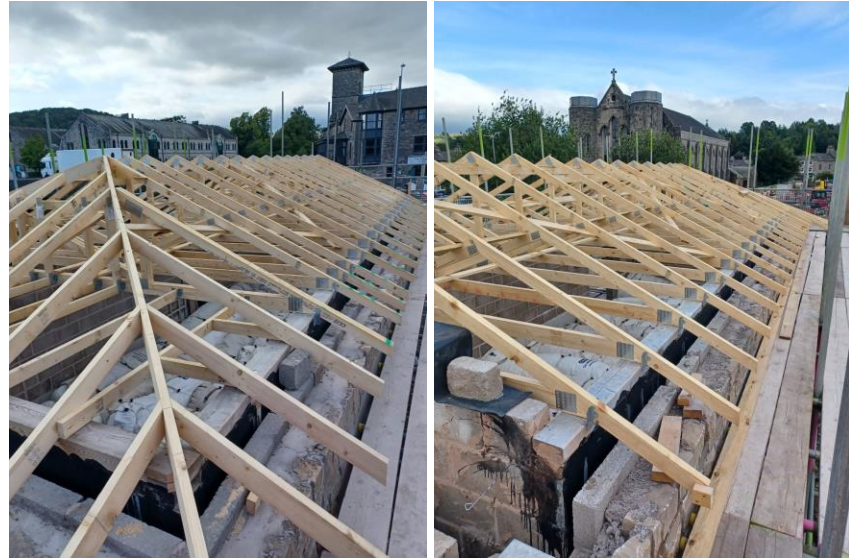
Motor Control Centre Building – Housing for all the electrical equipment for the Stock Beck pumps
