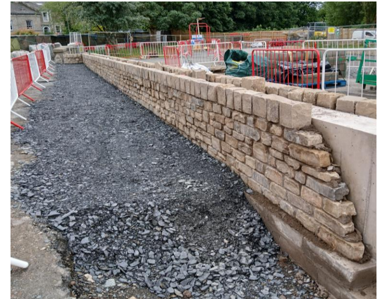
Floodwall along St Georges walk in Construction
