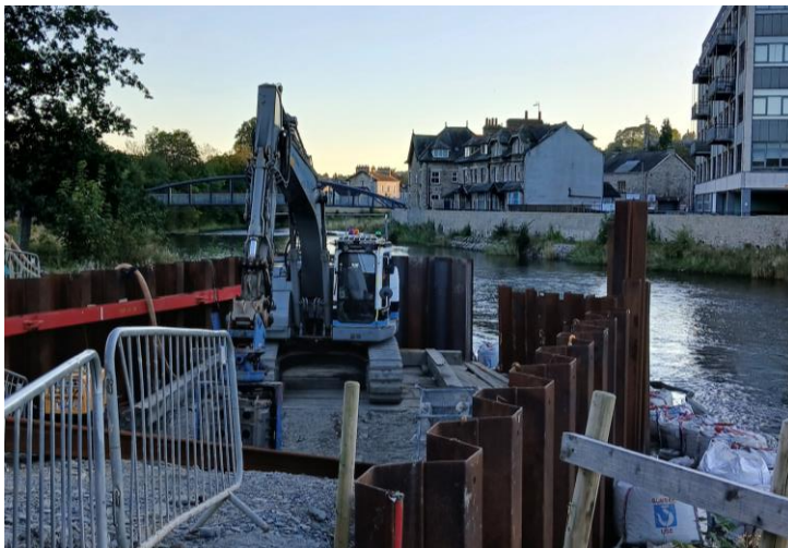
Outfall – The new outfall of Stock Beck into the River Kent.
