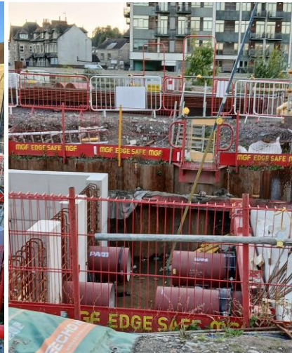
Valve chamber – Holding the pipe valves that pump Stock Beck onwards to the outfall
