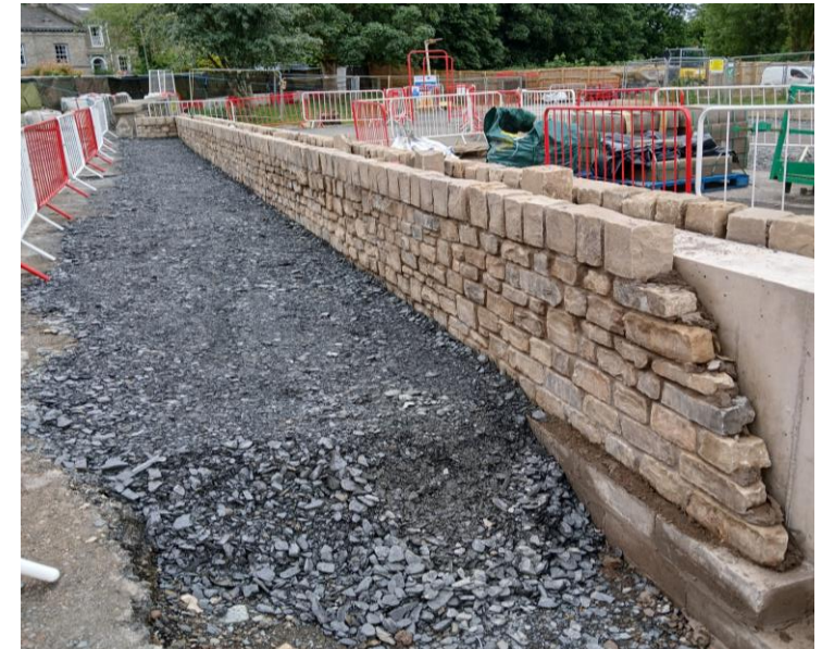
Floodwall along St Georges walk in Construction
