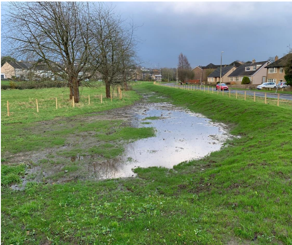
Image: View of surface water ponding along toe of flood embankment.
