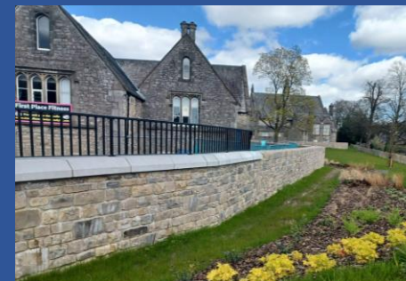
New flood defence wall around Kirkland Hall
