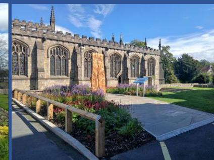
Flood wall and amphitheatre feature
