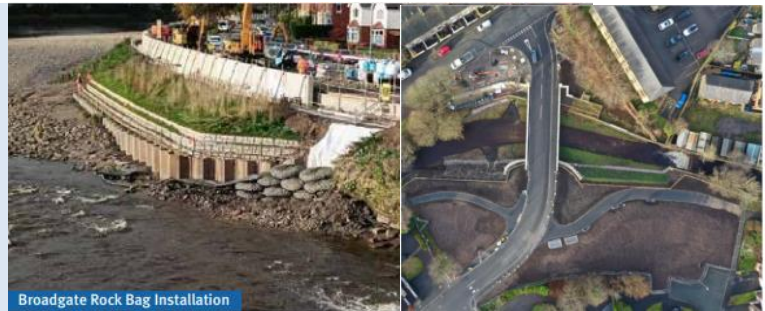
Broadgate Rock Bag Installation
