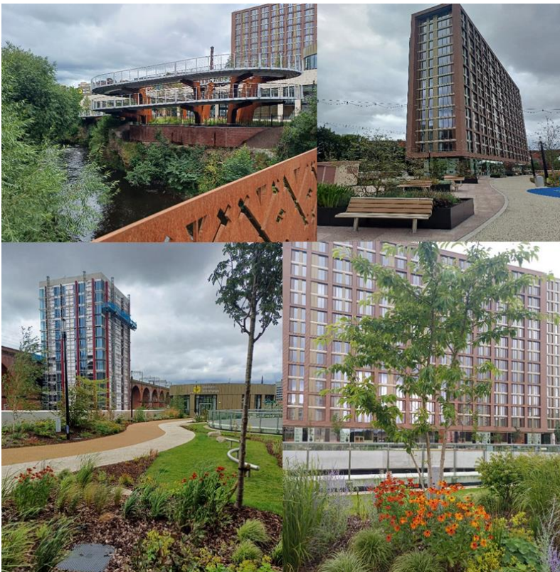
Figure 3: Stockport town centre interchange redevelopment
