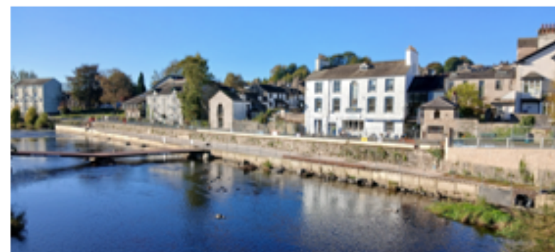
View of Waterside section which will benefit from a glass panelled flood wall.
