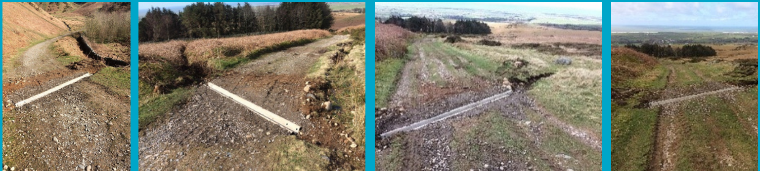
Images: West Cumbria Rivers Trust. Cross drains diverting runoff into surrounding vegetation
