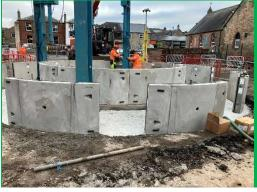
Left – Wet well, where the water will be collected and held, awaiting to be pumped into the river
