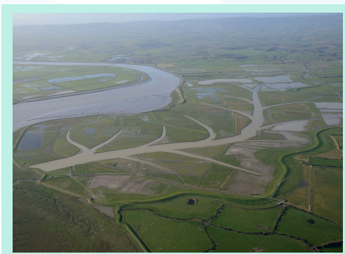
Image: Hesketh Out Marsh West in the Ribble Estuary during the construction phase -The Environment Agency
