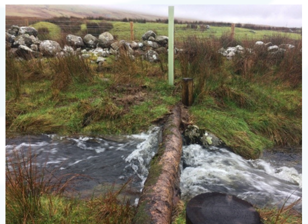
Image: West Cumbria Rivers Trust. Image of leaky dam
