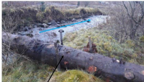
2 pins knocked in d/s, 1 pin knocked in u/s (pins are 2m long) and wired using high tensile wire. Notches were cut into pins to give wire a groove to sit in, to oppose upward force of water.
