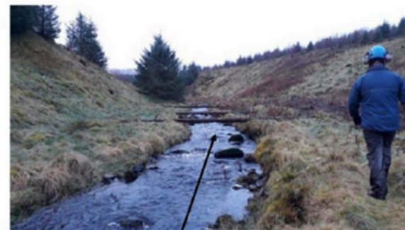
Locations of LWD features chosen due to topography and ease of access, taking advantage of floodplain width, bank height and what the machinery could easily move.
