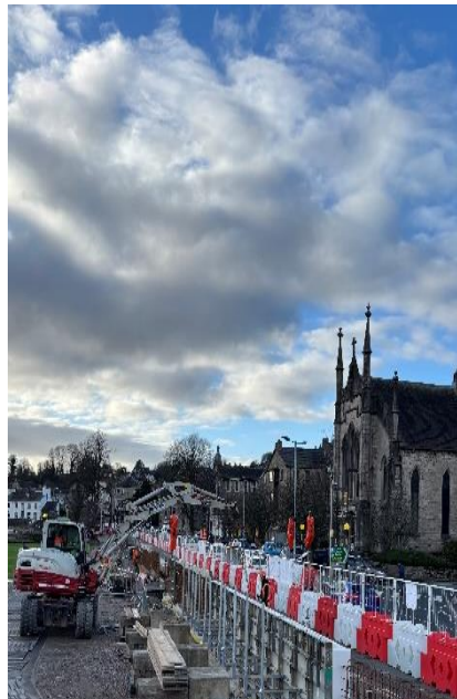
Flood wall in construction
