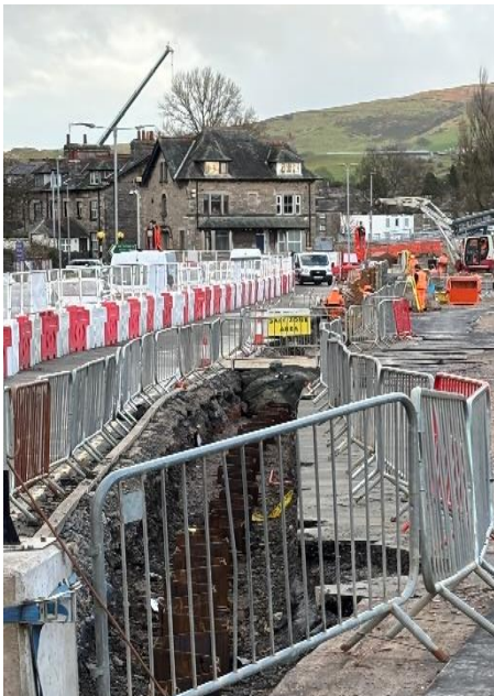
Sheet Piles in place
