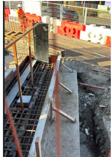
Flood gate foundations
