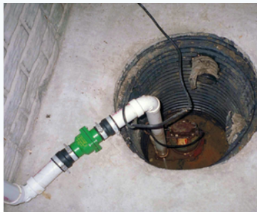
Image: Sump pump/ State Farm/ 13249921583 CC BY 2.0
