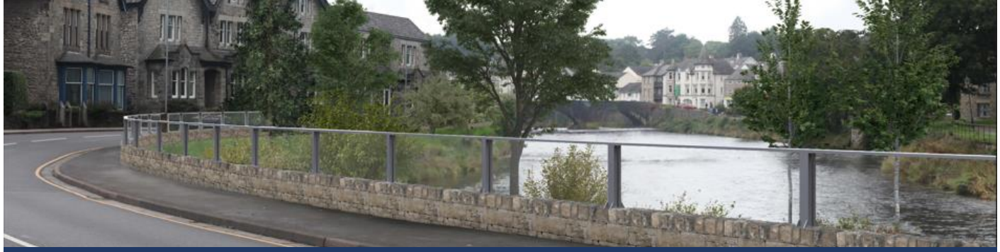
Aynam Road – Flood wall featuring slimline glass panels retaining and maximising riverside views
