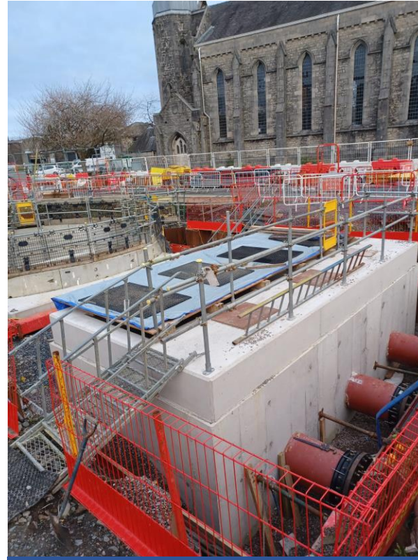
Valve Chamber undergoing pressure testing
