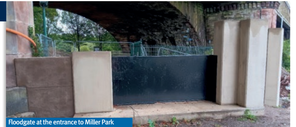
Floodgate at the entrance to Miller Park
