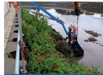
Rockbags being installed at 1B
