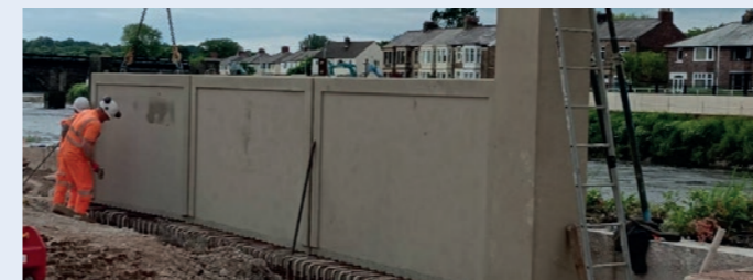
Construction of the new flood wall at Riverside Road has commenced
