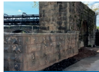
Local concrete artist's carving and paint work at the gas pipe bridge
