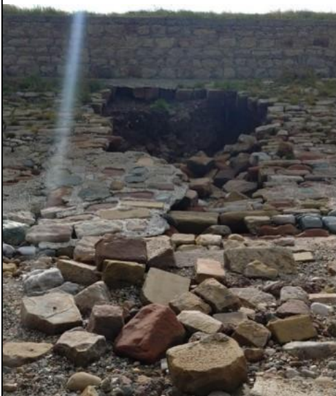
Image 2: Example of recent damage to raised defences at Thurnham
