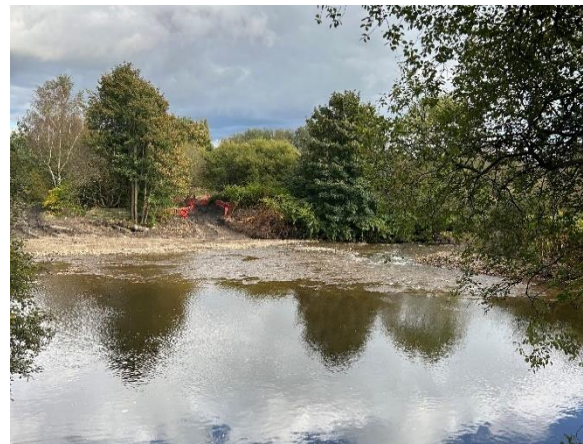
Hinds Weir After Removal
