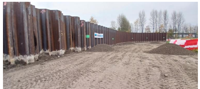
Piled wall beside railway line
