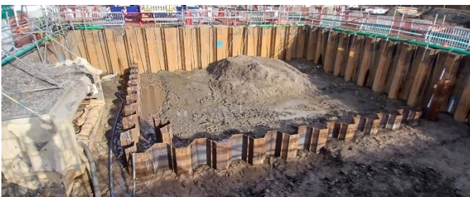
Gale East diversion structure cofferdam
