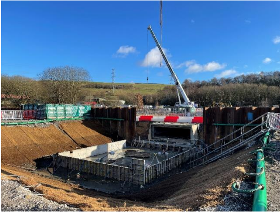
Extension of the culvert underneath the railway
