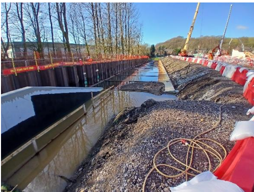
Completed reservoir spillway structure
