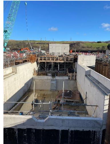
Gale West reservoir outlet structure
