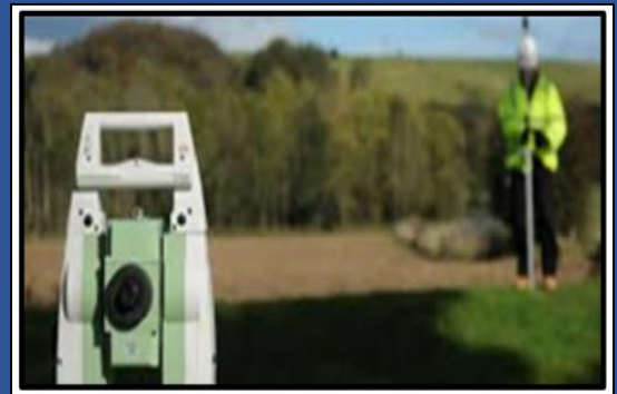
GPS laser and level equipment
