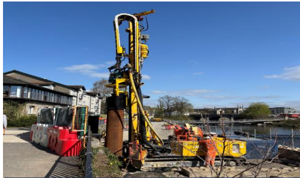
Piling using Spiral Flush method
