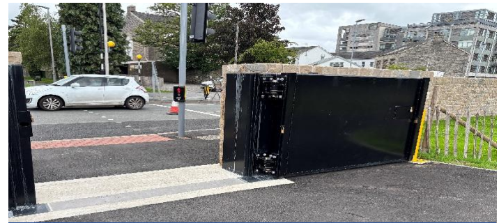
Flood gate at the pedestrian crossing
