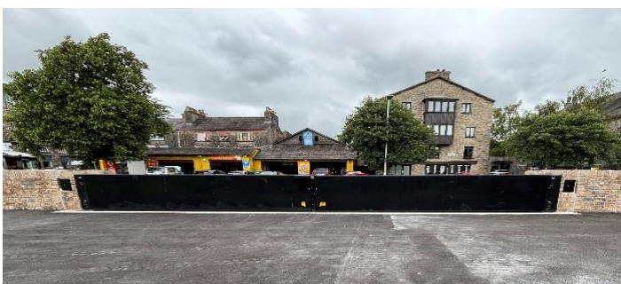
Large flood gate leading to the slipway
