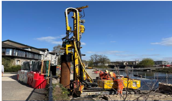
Piling using Spiral Flush method
