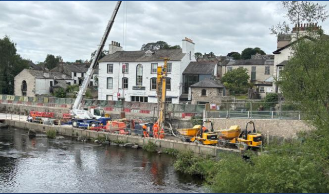
Piling continuing at Waterside
