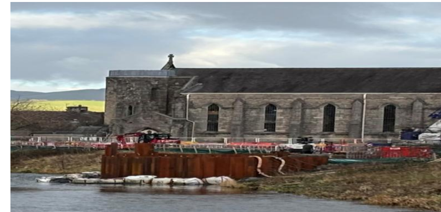
Piles of the cofferdam to be removed
