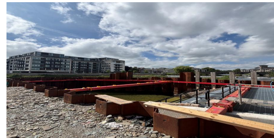
Frame & piles beginning to be removed
