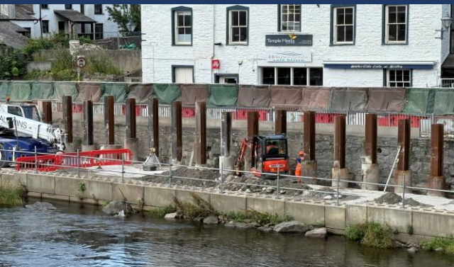
Inserting of king posts at Waterside
