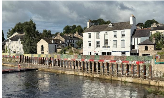
Platform with king posts inserted
