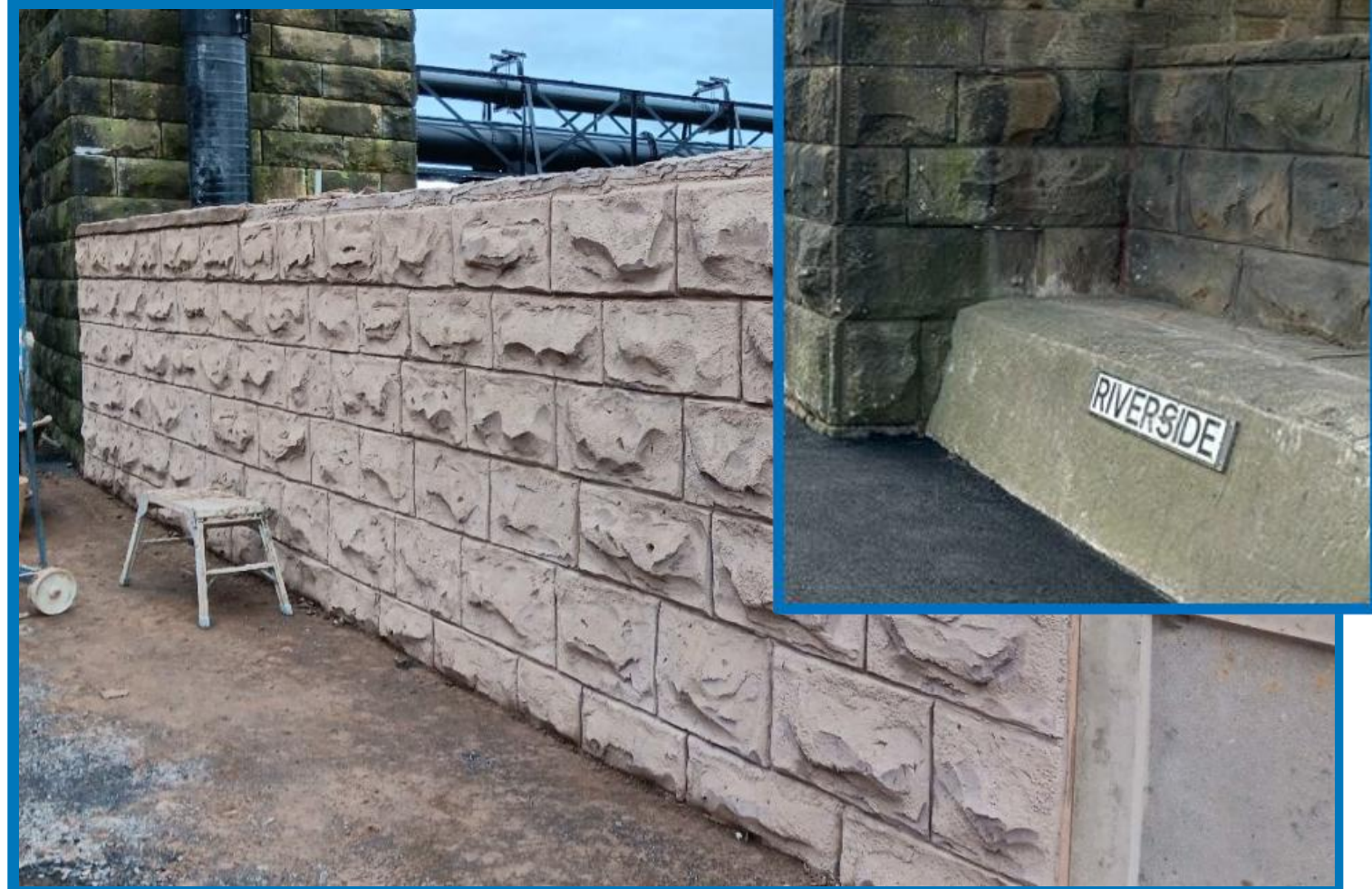
Concrete carving underway to blend a section of new wall into the Gas Pipe Bridge
