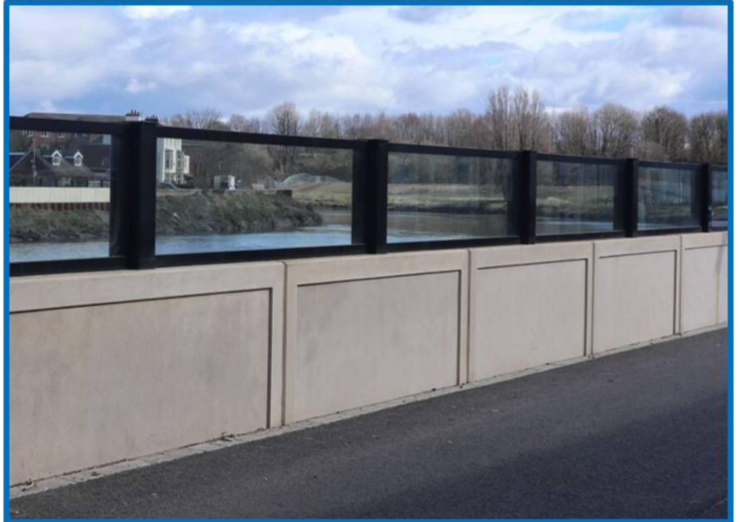
The new flood wall and glass panels along Riverside Road, Lower Penwortham
