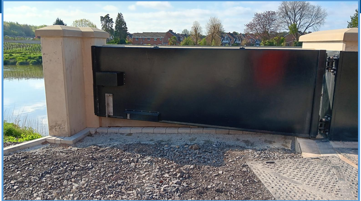
New floodgate under construction near Miller Garden Apartments
