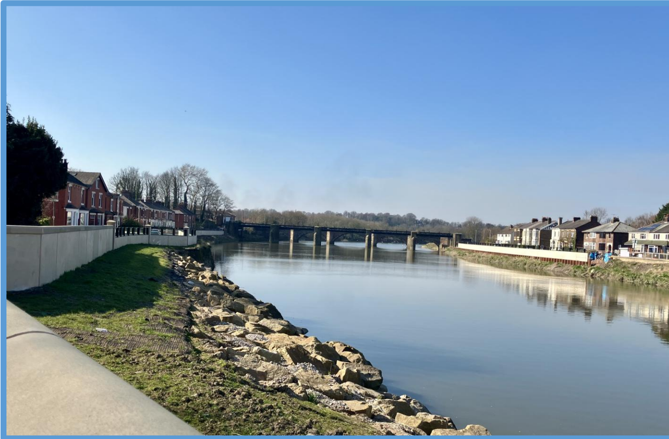
Rock armour along Riverside Road, Lower Penwortham
