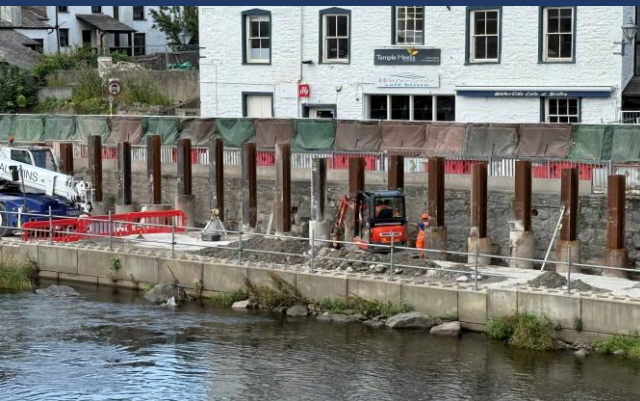
Inserting king posts at Waterside
