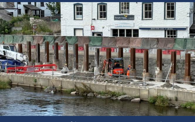
Inserting of king posts at Waterside
