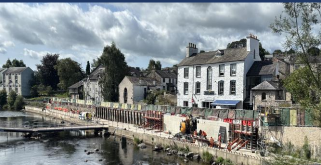
Construction of the flood wall at Waterside
