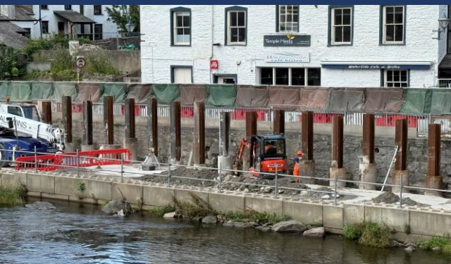
Inserting of king posts at Waterside
