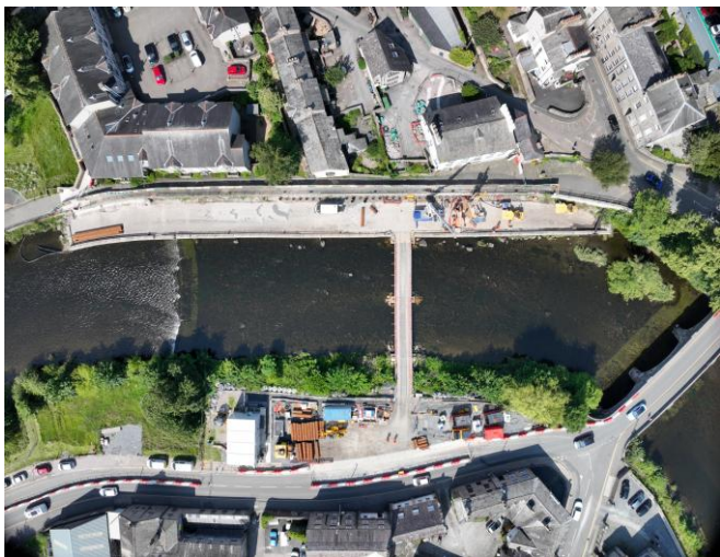
Aerial view of Waterside platform working area
