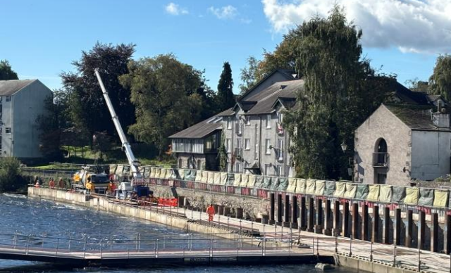
Inserting of king posts downstream at Edgecombe Court
